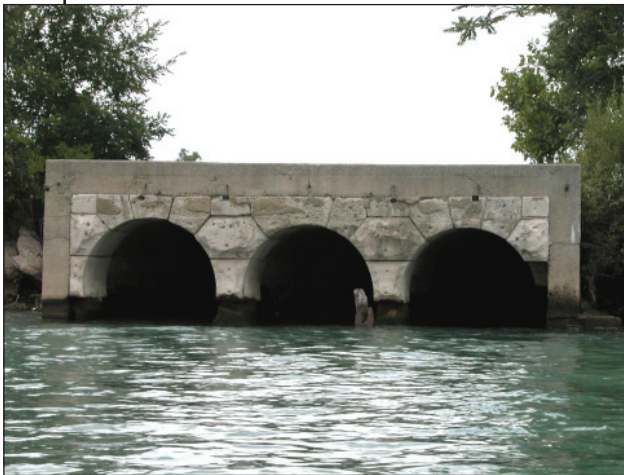
Figure 2. Combined sewer overflow outfall along the Detroit River (Photo credit: Robert Burns, Detroit Riverkeeper).
